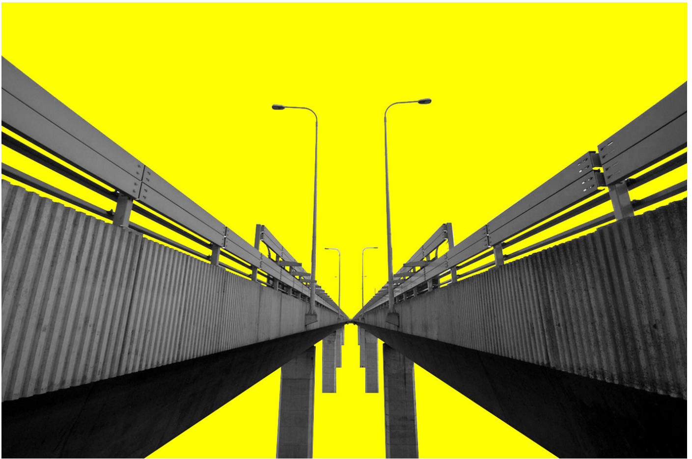
Figure . 5 - West link bridge cuts through the escarpment of the city formed by a river valley
